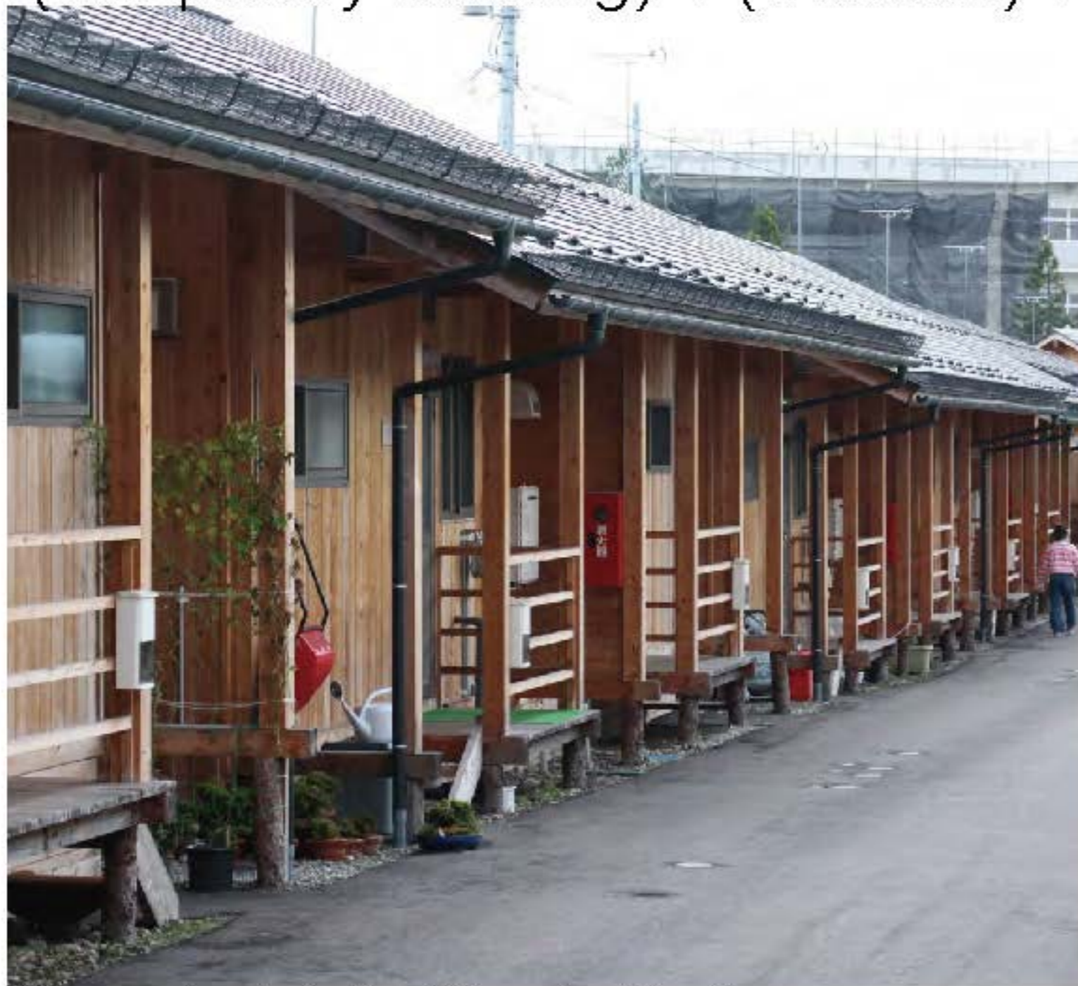
Temporary housing in Aizu Wakamatsu, Fukushima
