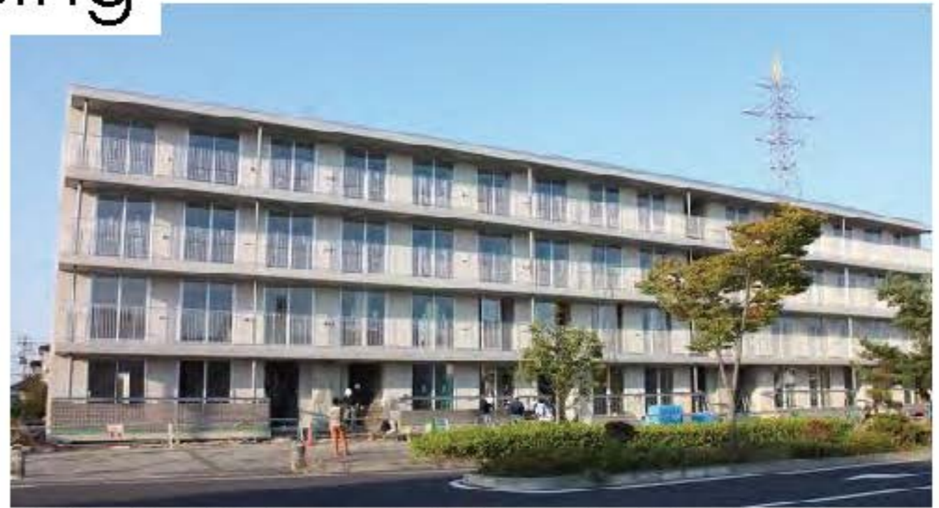
Multifamily public housing in Koriyama City, Fukushima
